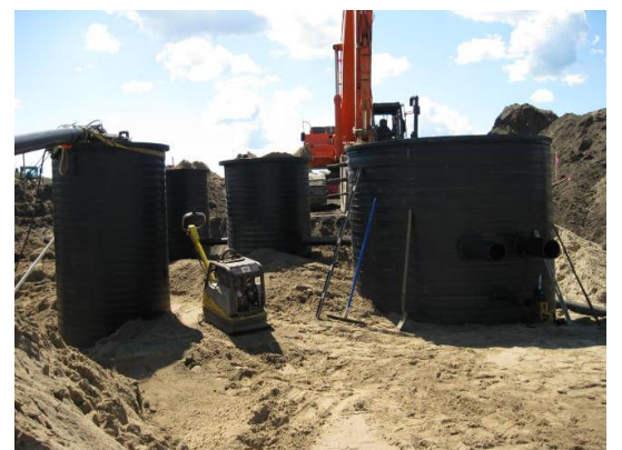
Construction of gap cell leachate pump at Solid Waste
