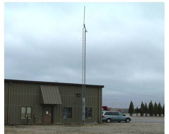
Transmission tower at Wastewater
