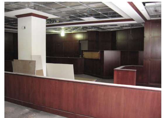
Courtroom construction at the Hall of Justice
