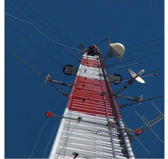
Installation of anemometers at nearly 400 feet
