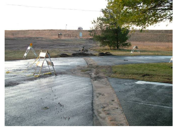
Pipeline replacement at the Wastewater Administration building
