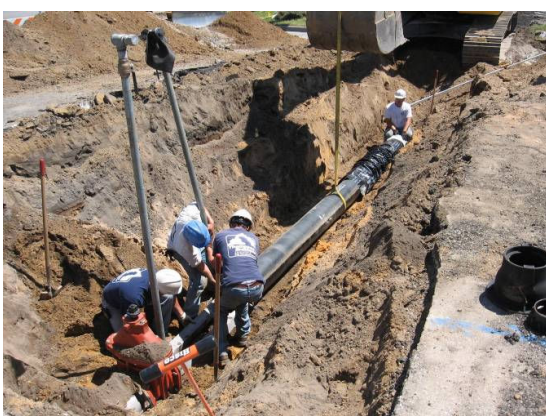
Great Lakes Ford water main extension
