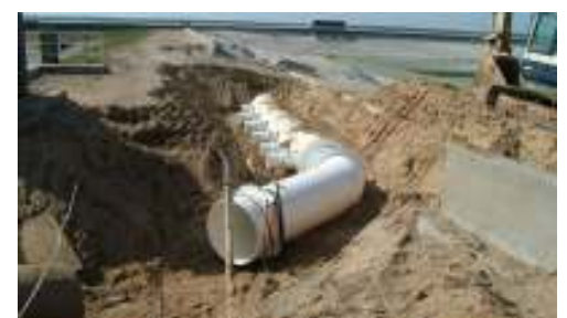
New header pipe for Pump Station #3 to allow room for strainers
