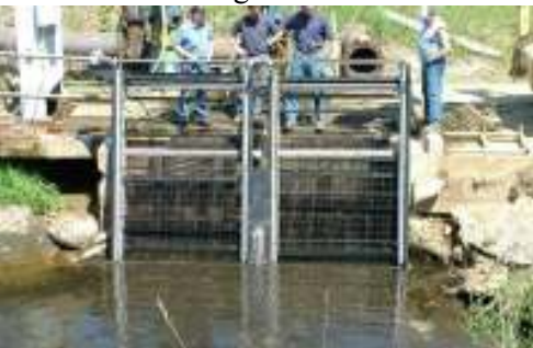
The rebuilt Sullivan Station trash rakes were installed this week
