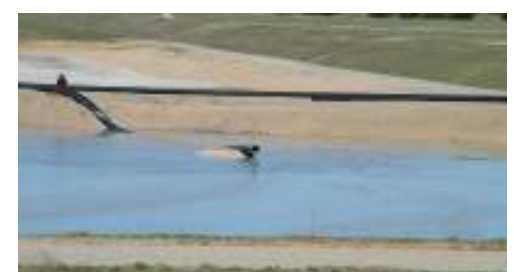
Sludge being pumped out to one of our drying beds at the Wastewater Plant
