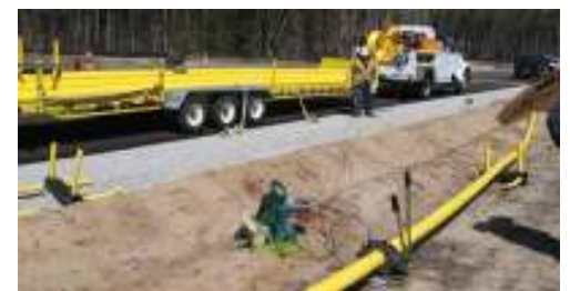
Natural gas lines being installed at our Business Park North
