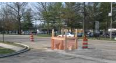
Access pit on Quarterline for installing the water main lining
