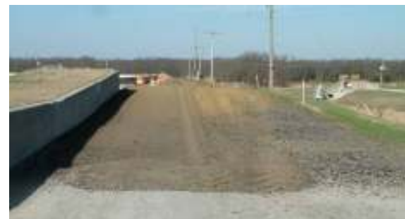
Roadbed preparation around Cell #1 where the flume was removed
