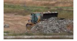
Stockpiling drying bed sludge
