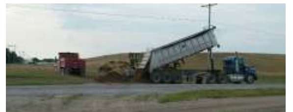
Gravel road improvements to Field 37
