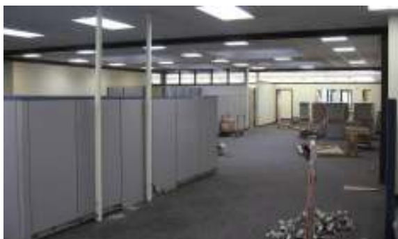
Office space progress inside the rebuilt "T-ROD" Building
