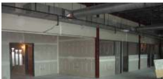
Drywall installation inside the new Halmond Center addition
