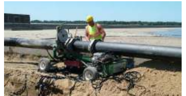
Fusing together the permanent sludge line under the Cell #3/#4 access area
