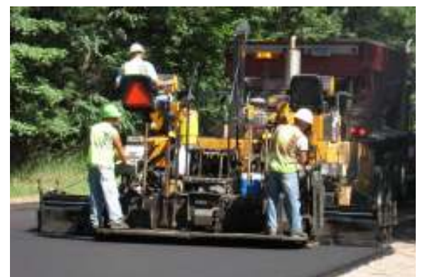
Paving Pennsylvania Avenue on Laketon Township Project
