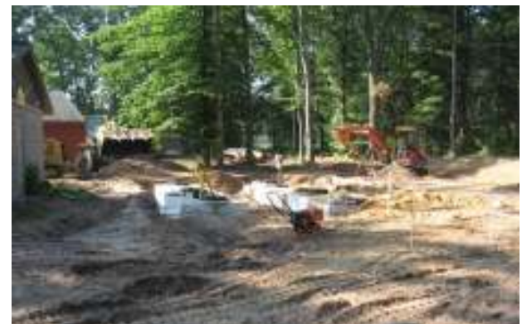
Septic system being installed at fairgrounds
