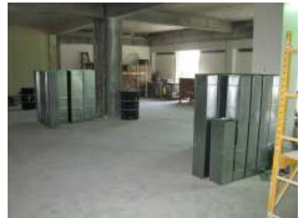
New steel ducting for Hall of Justice second floor
