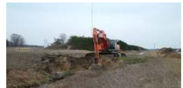
Emergency replacement of 60-inch culvert in main drainage ditch
