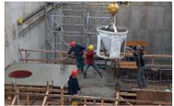
Pouring bridgework within the new Lift Station C dry well
