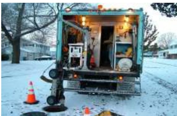
Contractor cleaning the Ruddiman Area Interceptor of roots and debris
