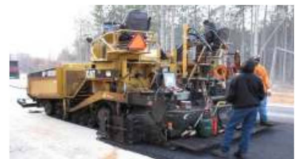
Paving work at our Business Park North
