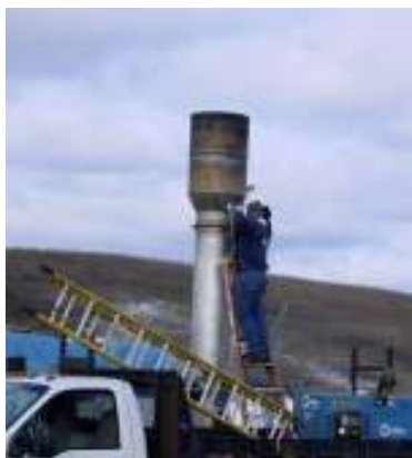
Contractor welding the pilot light in the landfill flare unit
