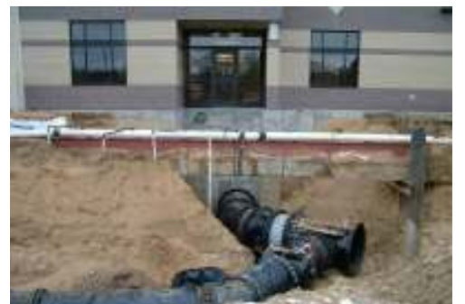
The new Lift Station C discharge piping was installed this period
