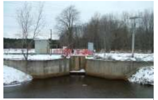
Laketon Station will be rebuilt to pump water to the RI or east storage lagoon
