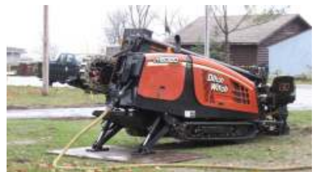
Directional boring machine used to install the Greenridge residential water services
