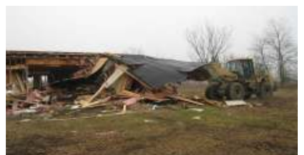
Demolition of Apple Avenue house
