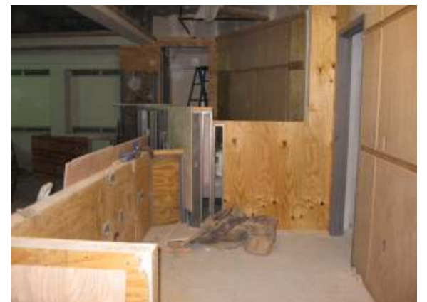
Framing work on a HOJ second floor judge's bench
