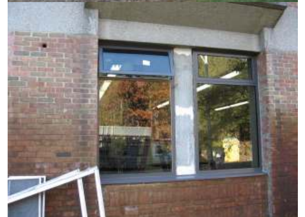
Window Replacement and Transite Panel Removal Energy Project at Brookhaven
