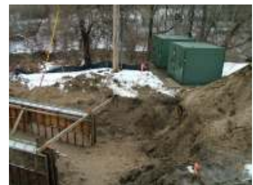
Forms for generator footing at D Station
