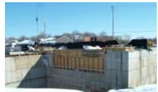
Above-ground concrete structure at new C Station
