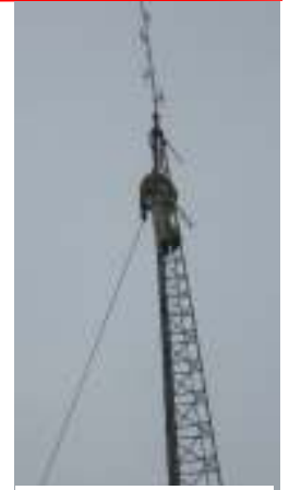
Water Tower radio cable replacement
