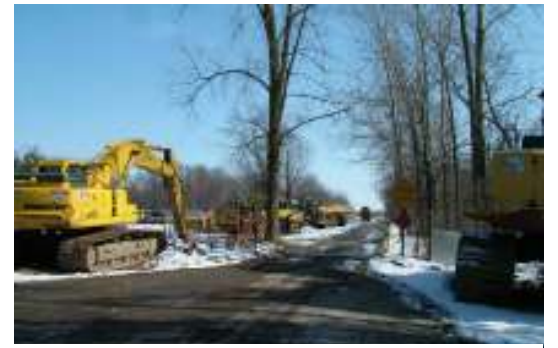
Contractor's equipment along Hall Road ready to lay pipe in March
