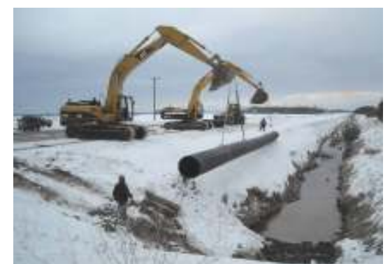
Lifting Swanson Road culvert liner into place
