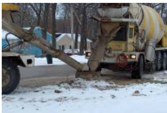
Pouring concrete in the abandoned 66-inch force main on MacArthur Road
