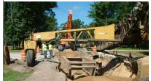
Jackson-Merkey Contractors laying 60-inch pipe on Marquette Avenue
