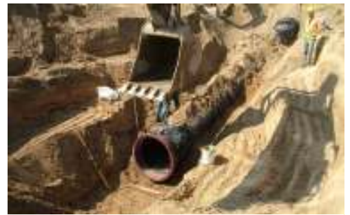
New force main pipe being laid at Cell #1
