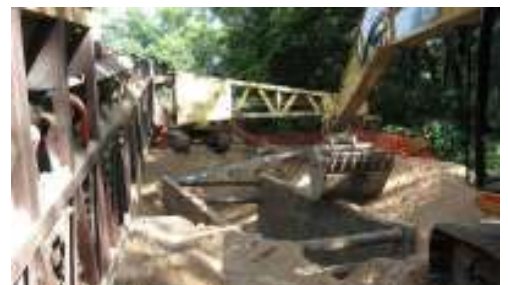
Sewer installation on Judy Lane in Laketon Township
