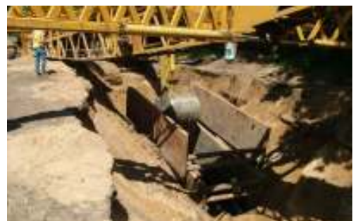
K&R on Hall Road placing 60-inch pipe 22 feet deep
