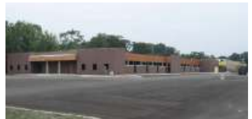
Halmond Building Addition
