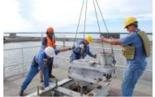
Operations Maintenance removed several mixer motors and gearboxes from Cell #2
