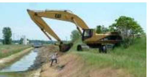
Max Rutz helps Ron Glover excavate the irrigation ditch side slopes
