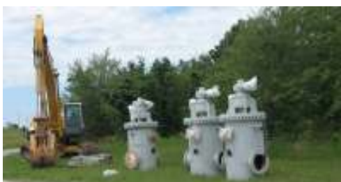
Large strainers for Pump Station #3
