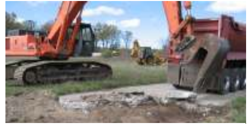
Removing concrete slabs at Business Park North
