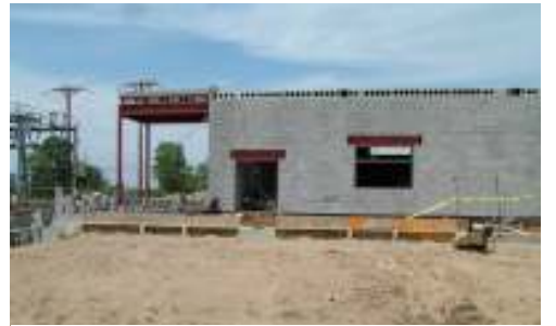
New Lift Station C construction
