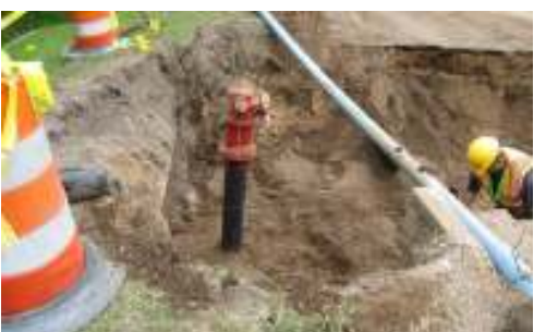
Hydrant installation on the Quarterline Road pipe lining project
