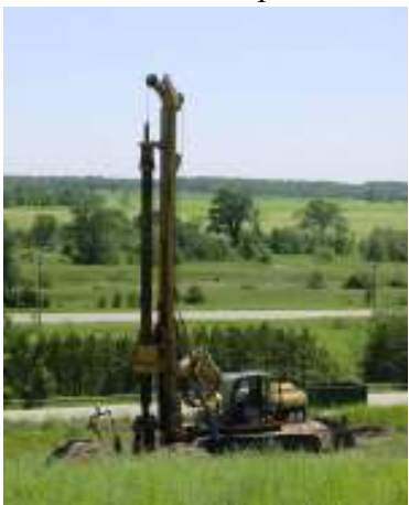
Drilling new gas wells at Solid Waste
