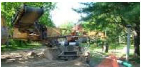
66-inch force main replacement near Marquette Avenue and Dangl Road
