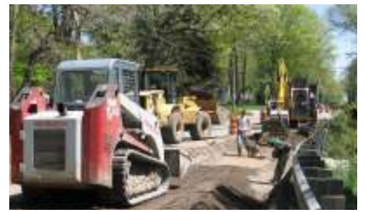
Sewer Force Main installation on Dykstra Road in Laketon Township
