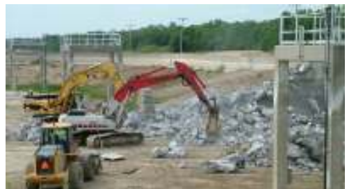
Demolition of the Cell #1 Pre-Aeration Chambers
