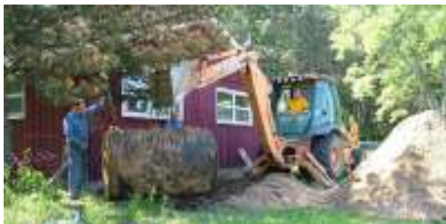
Fuel Oil tank removal at Whitehall Plant
