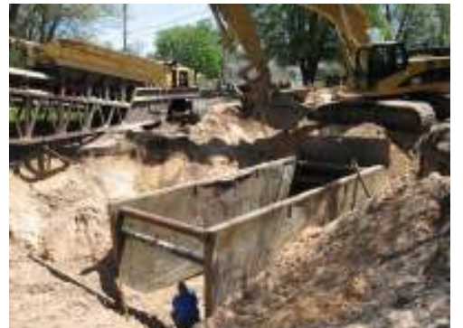
Gravity Sewer work on Memorial Drive in Laketon Township
