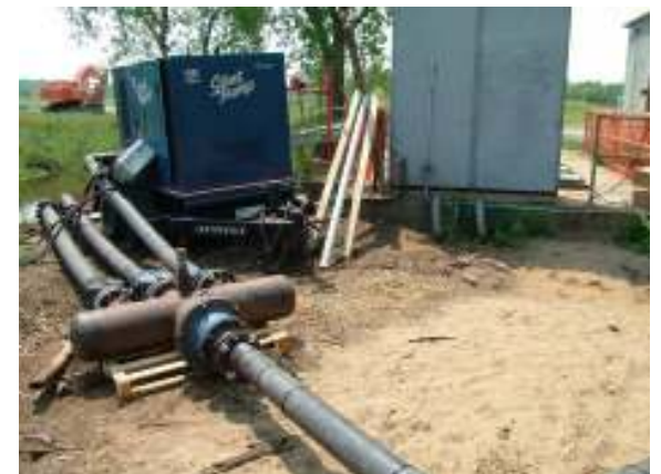
Bypass pumping at Laketon Station
