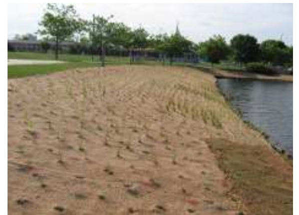
Heritage Landing bank restoration with mulch blankets and native grass plantings
