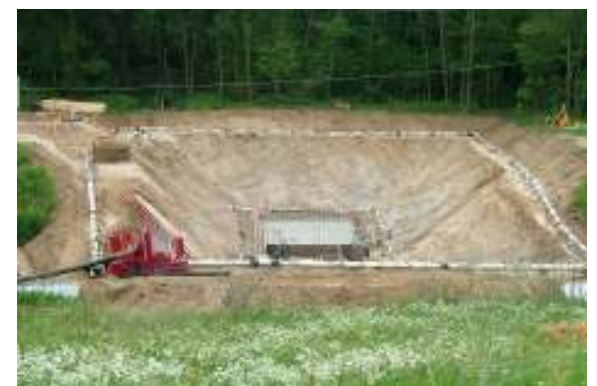
Base slab poured for new Sullivan Station
