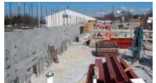
Block wall going up at Lift Station C
