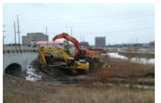
Construction on C Station Overflow at Ryerson Creek
