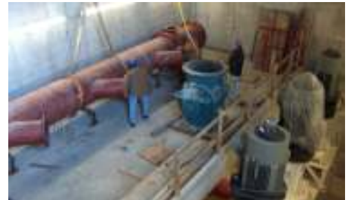
Lift Station C pump header being installed
