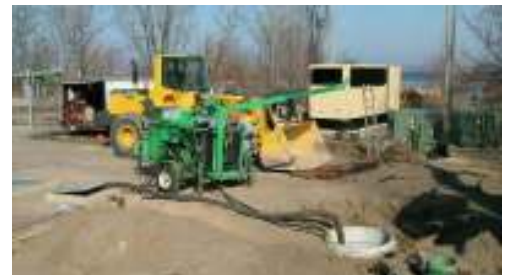
Demolition of the old 1973 vintage Lyco Lift Station D
