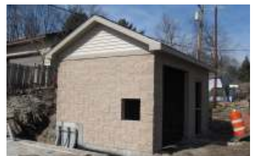
Horton Road sewage lift station in Laketon Township
