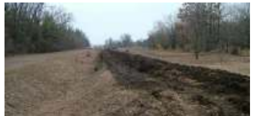
Partial clearing of pipeline route along east side of Sullivan Road
