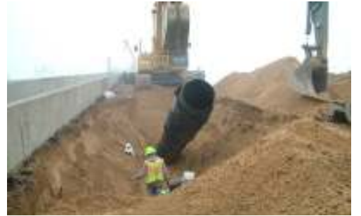
Laying pipe south of Cell #1
