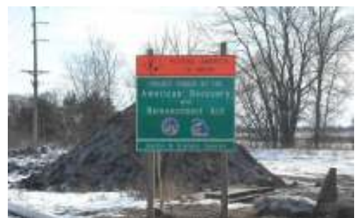
Station/pipeline project is being partially funded by ARRA principal forgiveness
