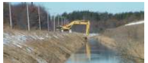
Cleaning lagoon interception ditch with wastewater excavator
