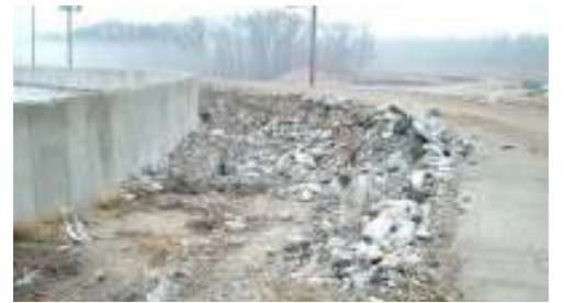
Demolition of flume around Cell #1
