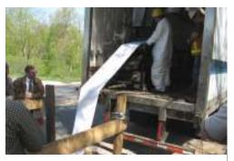
John Warner observes liner being placed in water pipe on Quarterline Road
