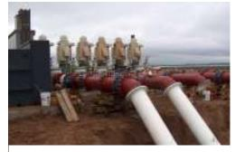
Pipe work at Pump Station #3 as part of the strainer addition
