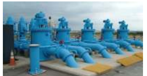
Pump Station #3 painting almost complete
