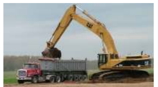
Loading sludge into one of Watts Trucks
