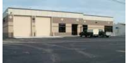
New parking lot paved at C Station
