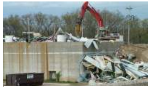
Demolition of Pre-Aeration Building
