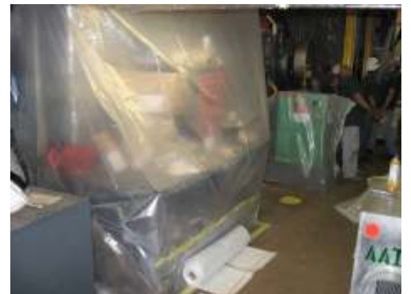
Hall of Justice asbestos removal prep work
