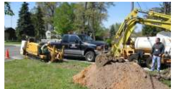
Residential water service installation on Memorial Drive in Laketon Township
