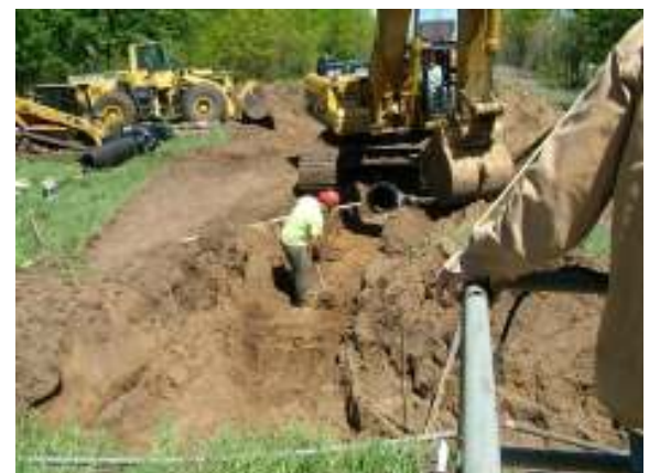
Pipeline almost completed to Laketon Station
