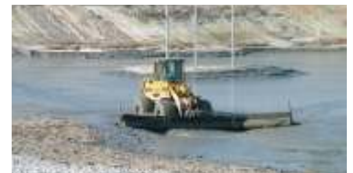
Contractor pushing sludge to be pumped out to the drying beds
