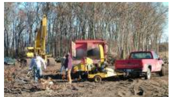
Chipping brush and small limbs from Field #7 clearing activity
