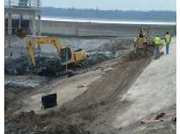
Laying 42-inch influent piping into Cell #2
