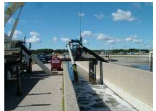
Pumping the water off the sludge in Cell #2
