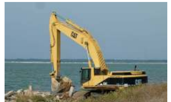
Removing the East Lagoon break water
