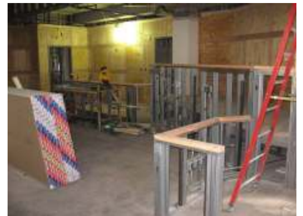
Drywall work at HOJ 2nd Floor
