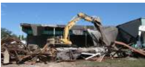
Warehouse demolition on our Business Park North site
