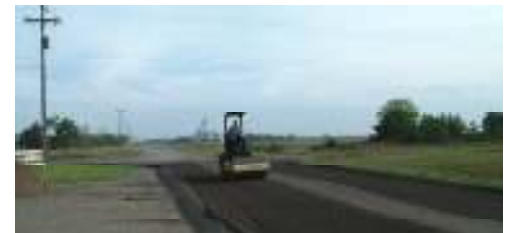
Recycled asphalt was put down as a roadbed at Wastewater
