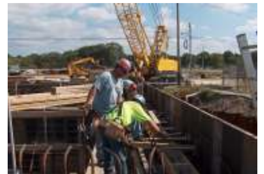
Tying steel at ground level at Lift Station C
