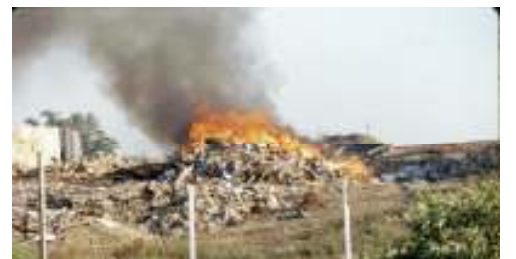
Demo materials on fire at Solid Waste
