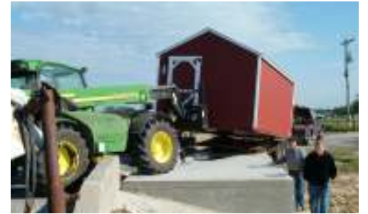
Installing our new hauled waste well house
