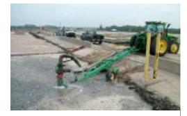
Pumping floating grease from Cell #3 to Cell #4
