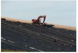
Landfill liner being placed on the east face of the "Gap"
