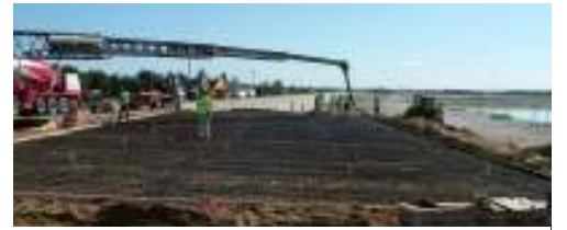
Pouring concrete for the hauled waste receiving area at Cell #4
