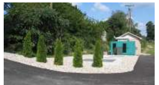
Another Laketon Township lift station near Green Creek
