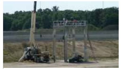
Setting Mixers in Cell #1
