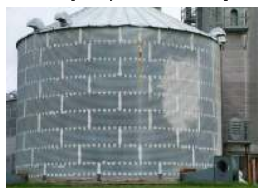
Painting in progress at the Grain Center
