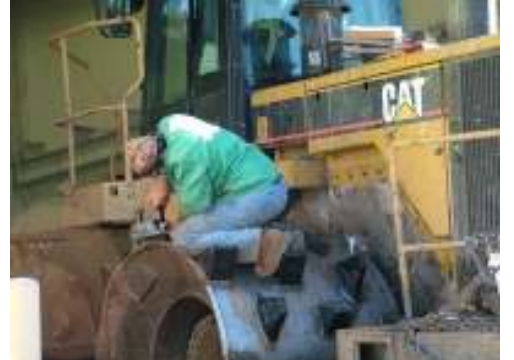
Contractor replacing one of the landfill compactor's spikes
