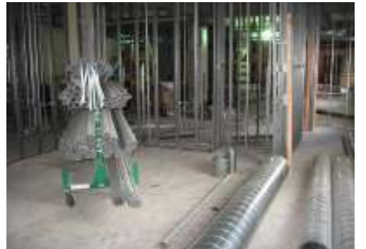
Steel wall framing at HOJ second floor
