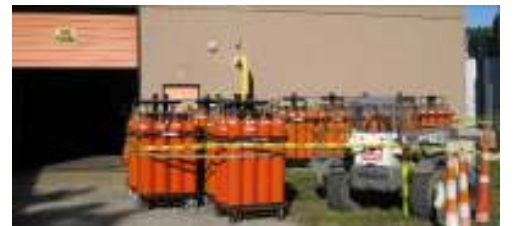
Nitrogen used to fill the waste gas line for testing at 100 PSI
