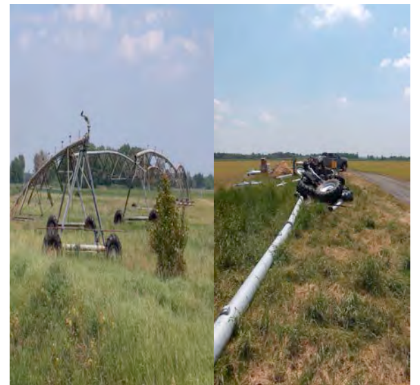
Dismantling of the worn out irrigation rigs
