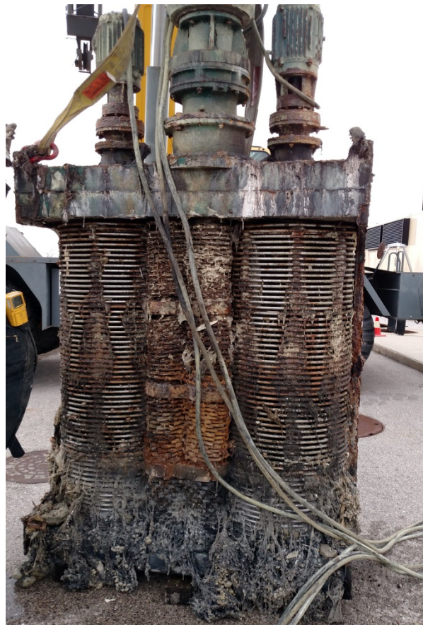
Old communitors being removed from C-Station.
