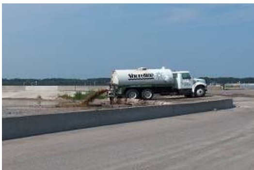
Figure 1 - Septic Hauler discharging into Cell #4
