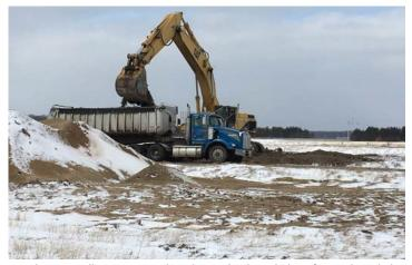
In February, Yellow Rose Trucking began hauling sludge from the sludge drying beds to the landfill after the Board of Public works awarded them the sludge hauling bid at the February Board meeting. The Wastewater's heavy equipment operator Chris VanderLaan is shown above using our excavator to load the trucks doing the hauling.
