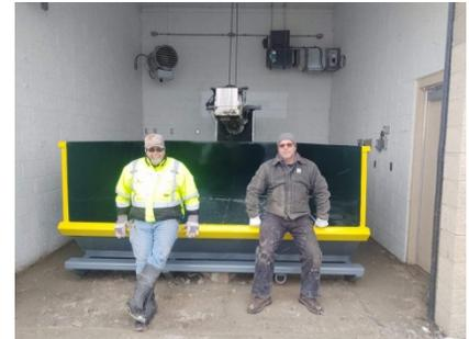
which allows a telehandler bucket to get in and scoop out the screenings and haul them to one of our nearby sludge drying beds. Since installing the new dumpster, we've never had to shut down the bar screen due to an over-full dumpster, and we've cut expenses by discontinuing the dumpster pickup service. This screen system keeps debris out of the aeration cells which saves the aerators from plugging and saves our mechanics loads of work needed to clean a plugged aerator.
